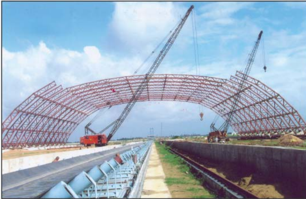
Coal shed under construction at Sagardighi
