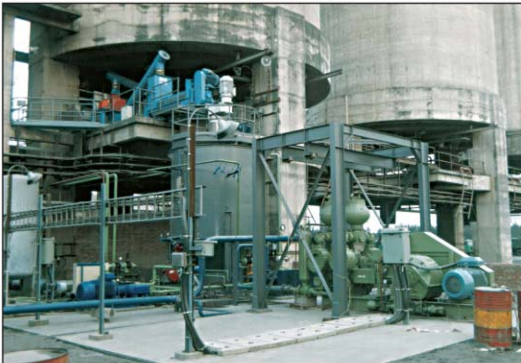
High Concentration Slurry Disposal System at CESC. Budge Budge
