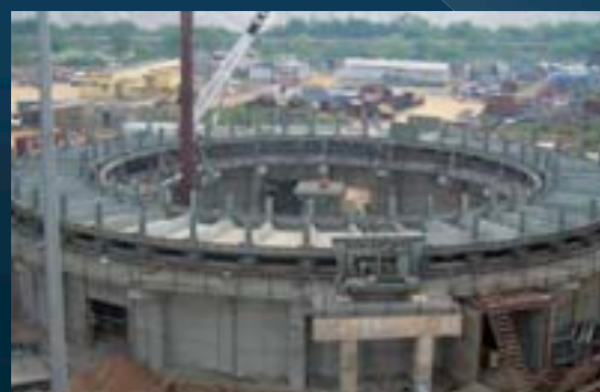
Circular Sinter Cooler (under construction)
